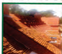
Handmade clay tiles roof in progress
