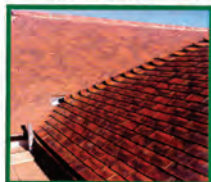
Handmade clay roof filling
