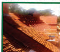
Handmade clay tiles roof in progress
