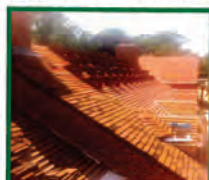
Handmade clay tiles roof in progress
